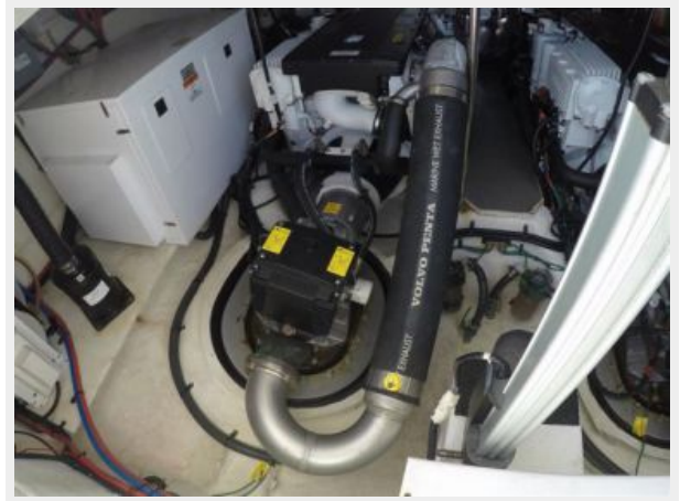
Generator w/sound shield
