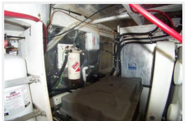
Forward view of Engine Room
