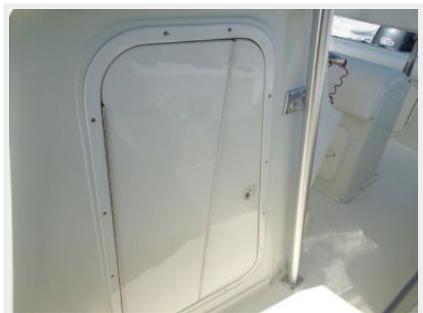
Door to Enclosed Head
