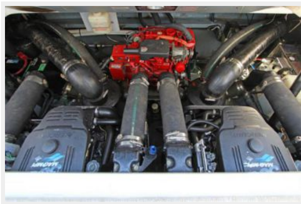
MerCruiser 350 MAG MPI Engines & Westerbeke Generator
