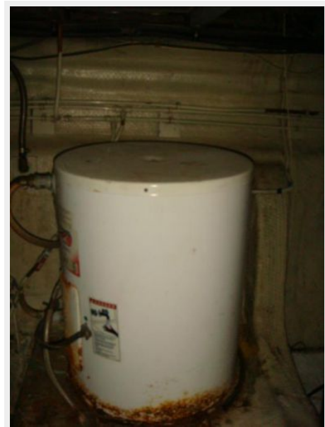
45' Chris Craft Water Heater
