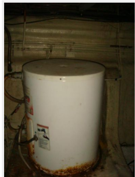
45' Chris Craft Water Heater
