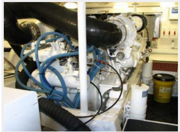
Engine & Mechanical Equipment 3 - Port Engine
