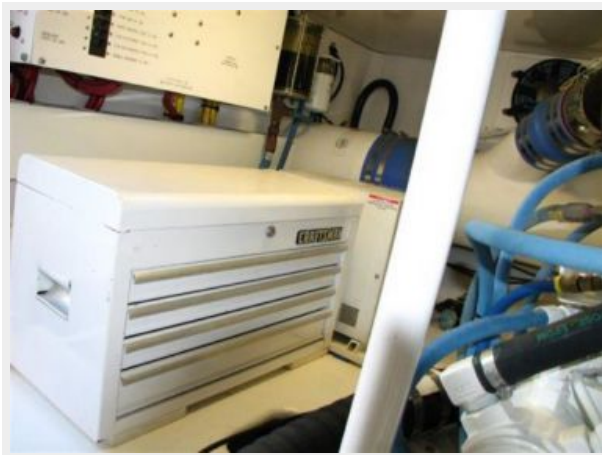
Engine & Mechanical Equipment 10 - Engine Room
