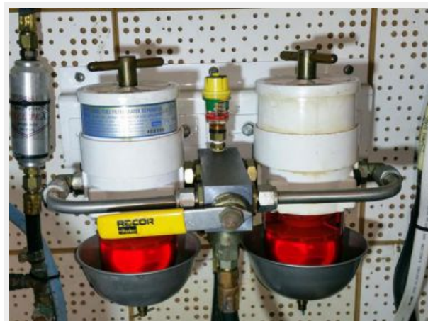
40' Albin Main Engine Racor Fuel Filters
