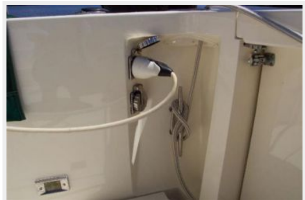
Dockside Electrical Connection
