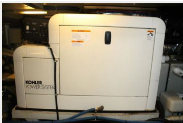
Generator Sound Shield
