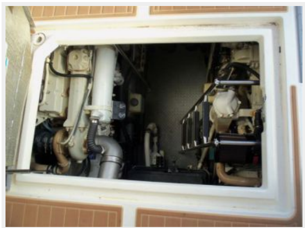
Engine Room Access
