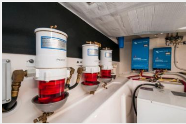
Raycors & Battery Charger
