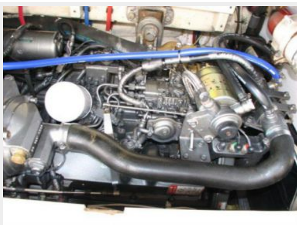
Engine & Mechanical Equipment 2 - Starboard Engine
