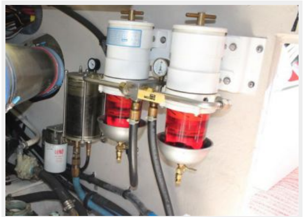
Starboard Dual Racors with Pressure Gauge
