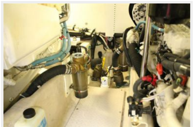
Clean Bilges & Raw Water Strainers
