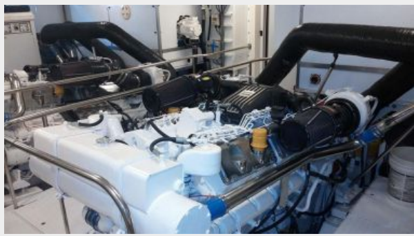
Engine Room Port Side
