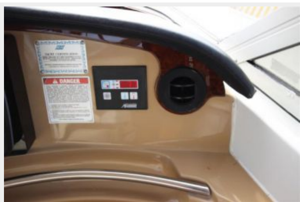
Helm Bridge AC
