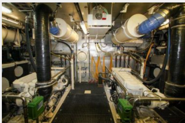
Engine Room Forward
