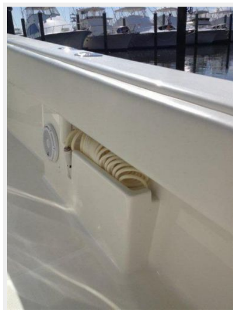
Deck 5 - Salt Water Wash Down
