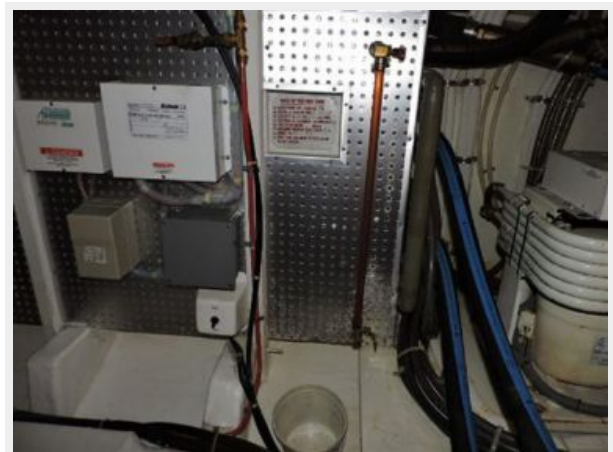
Fuel Tank and Site Gauge
