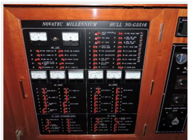
Shore Power Panel
