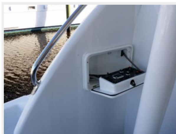
Aft Control Station
