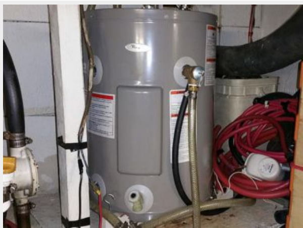
49' Marine Trader Water Heater
