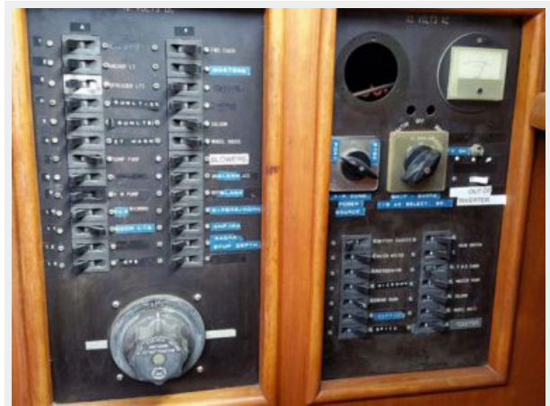
49' Marine Trader Electrical Panel
