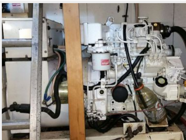
49' Marine Trader Generator
