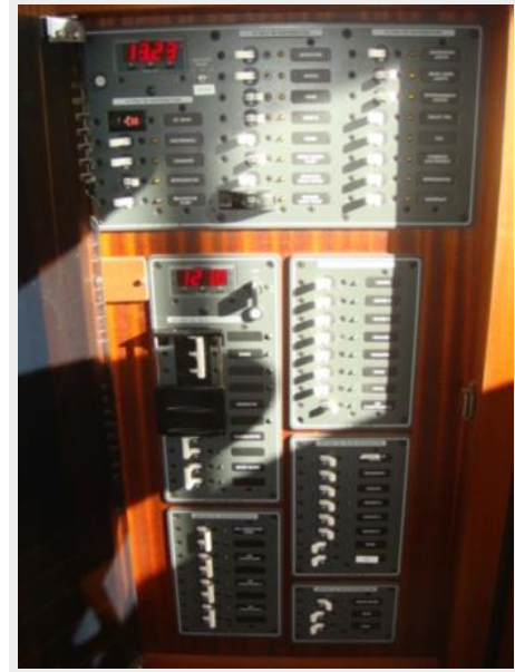
41' American Tug electrical panel
