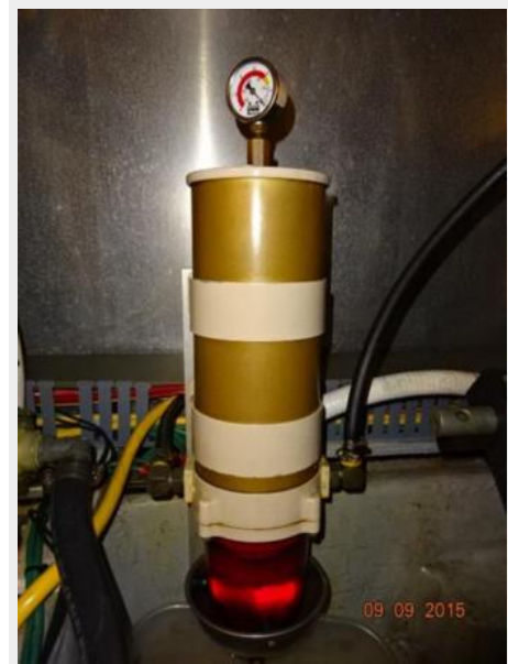
43' Mainship starboard Racor fuel filter
