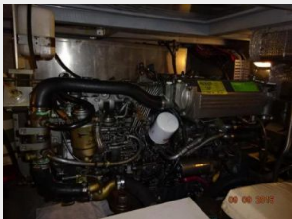
43' Mainship starboard main engine
