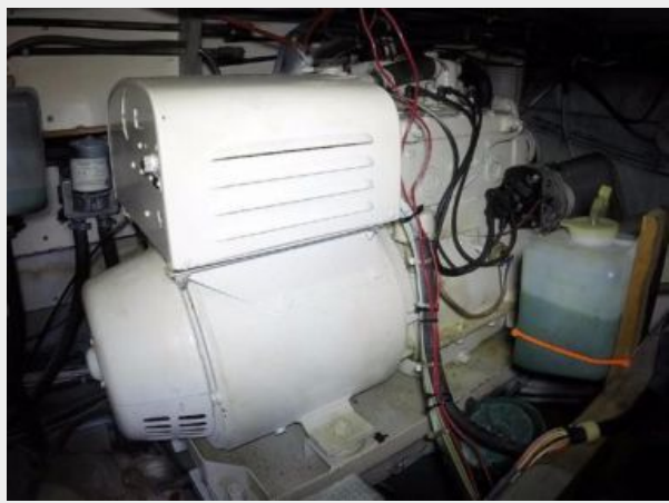
36' Chris Craft Generator
