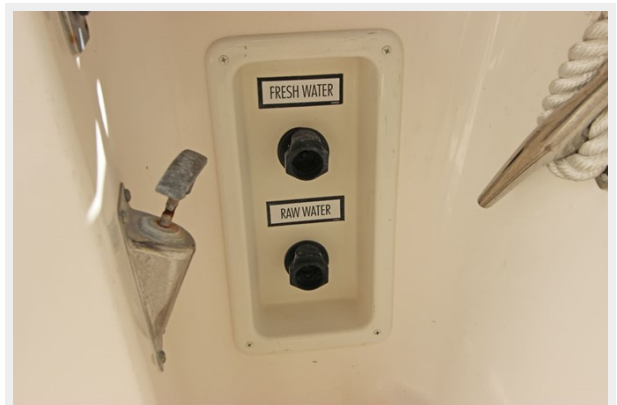
FRESH & RAW WATER WASH-DOWN IN COCKPIT
