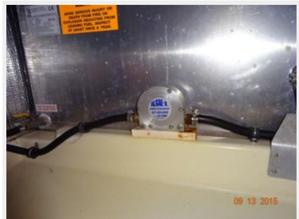
31' Camano Algae-X fuel conditioning system
