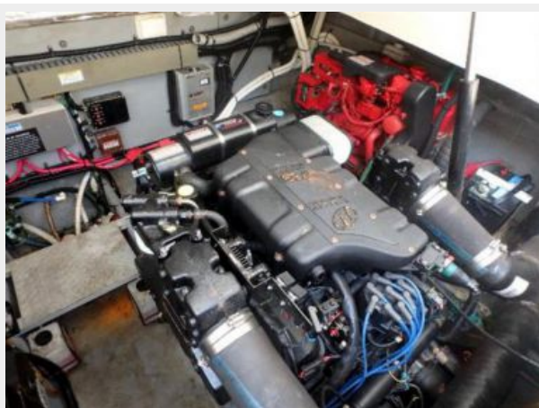
Engine Room II
