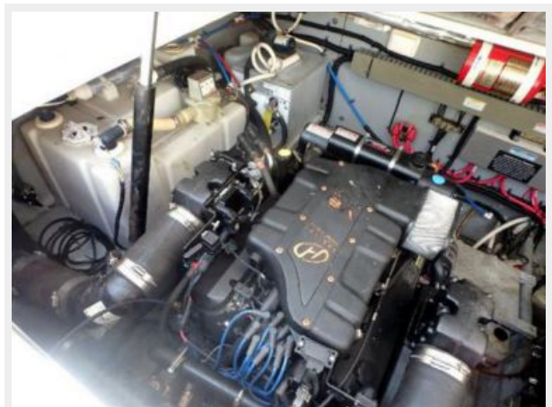
Engine Room III
