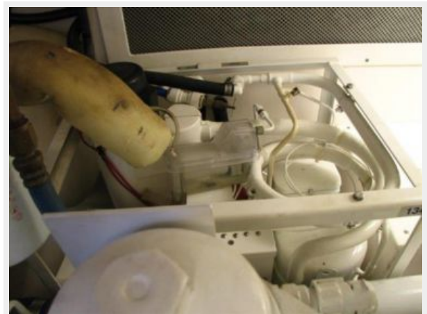
Engine & Mechanical Equipment 8 - Ice Chipper
