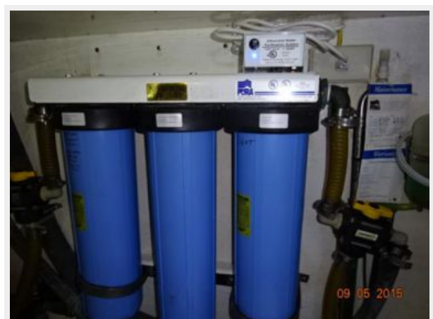
54' Ocean Alexander fresh water system filtration
