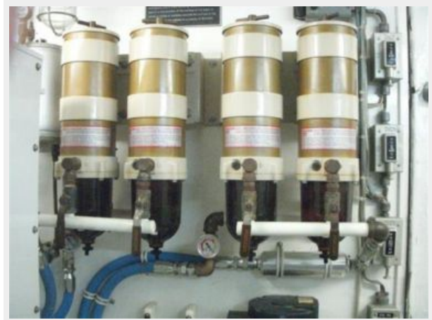
Racor Switchable Filters
