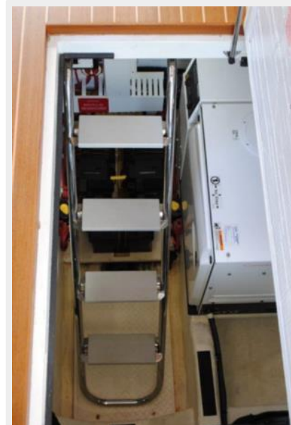
Engine Room Access
