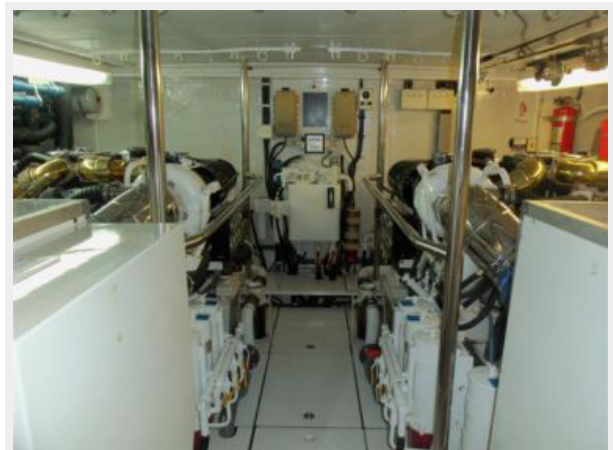
Engine Room Looking Forward
