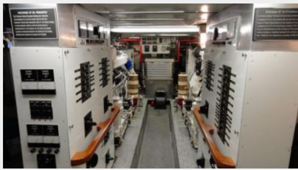
Engine Room Looking Aft
