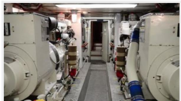
Engine Room Looking Fwd.
