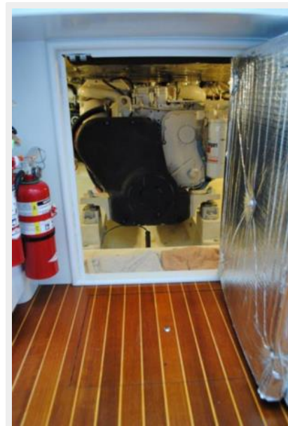
Engine Room Access
