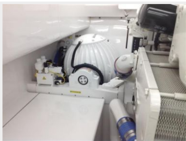
Engine Room - Seakeeper Gyro Starboard
