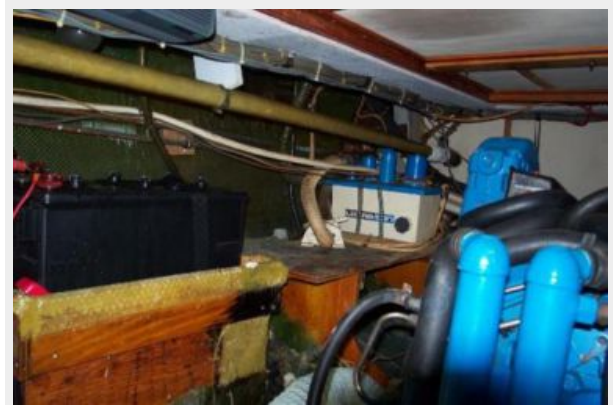
Engine Room-outboard, starboard
