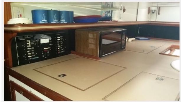
Counter below Companionway
