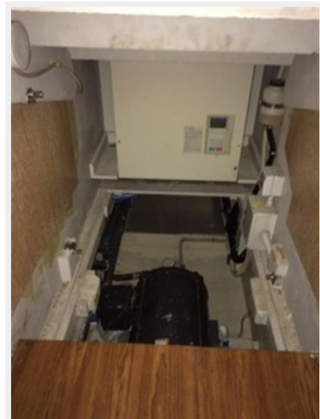
Entrance to Lower Level Mechanical Tunnel
