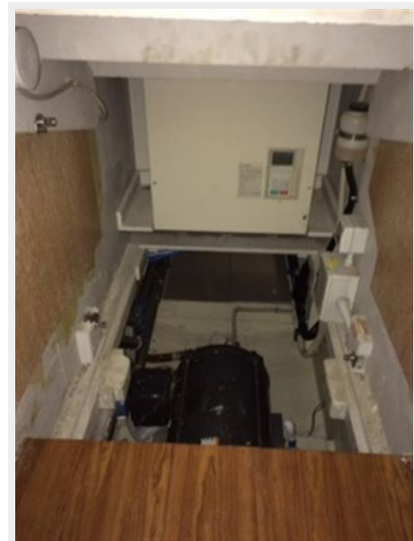
Entrance to Lower Level Mechanical Tunnel
