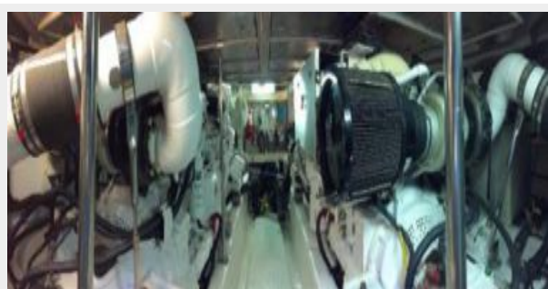
Engine Room Looking fwd
