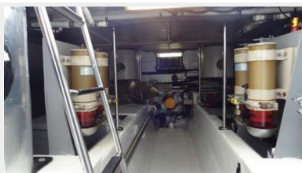
Engine room access
