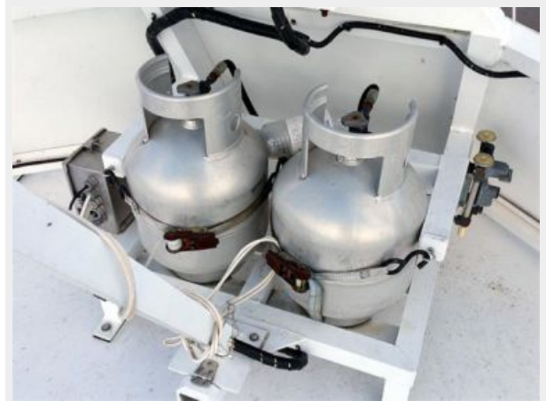
North Shore 34 Propane Storage
