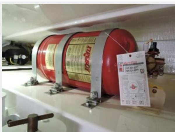
Fireboy Automatic Fire Extinguisher System
