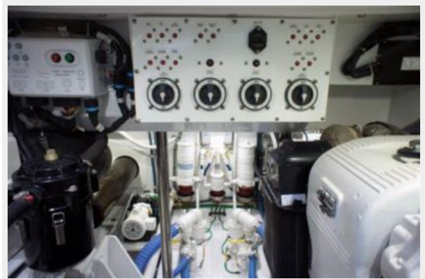
battery switches, racor filters, white painted thru hull fittings
