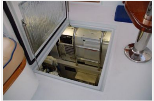
engine room entrance
