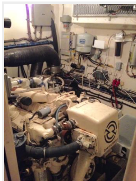
Port Engine Room
