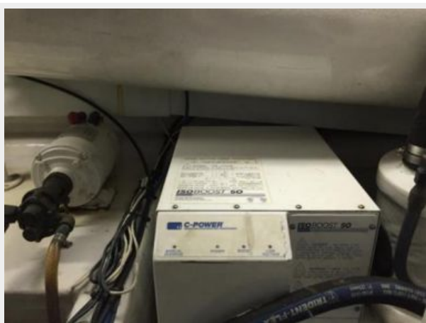
ISO Boost Isolator Transformer
