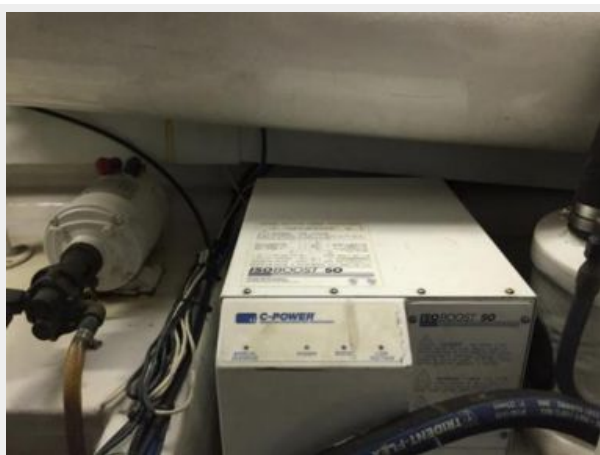
ISO Boost Isolator Transformer
