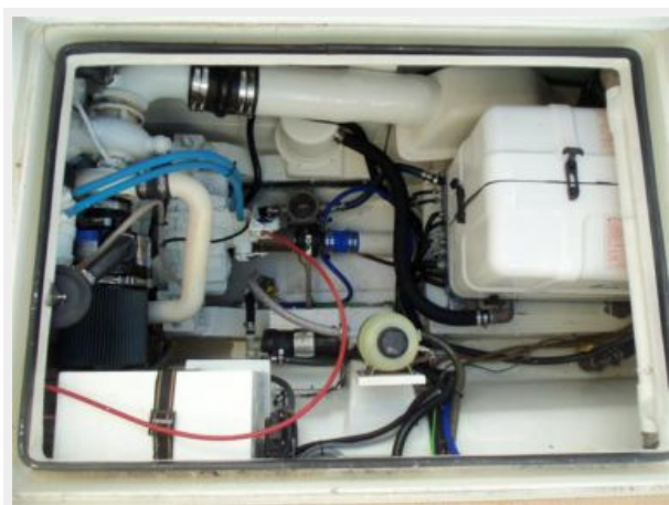
Starboard Engine Room Aft
