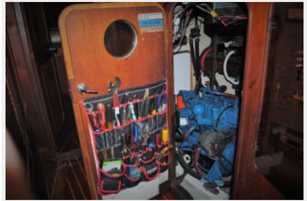
engine room door
